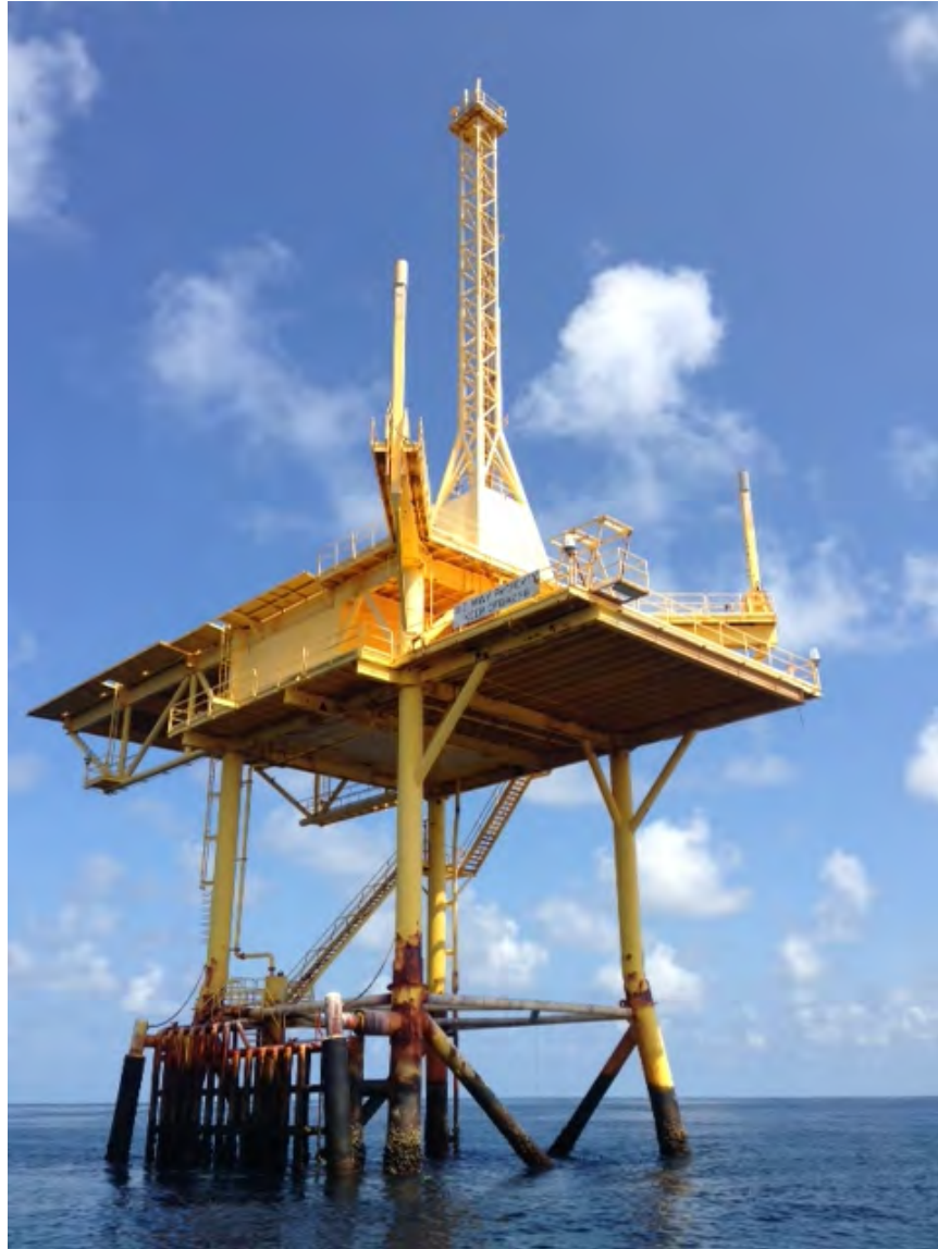
Figure 2.3: Abandoned Navy Tower R2 (31°22'30"N, 80°34'01"W) off the coast of Georgia. All three Navy Towers used in this study (R2, M2R6, and R8) are similar in design and size (Photo credit to Chris Briand).
